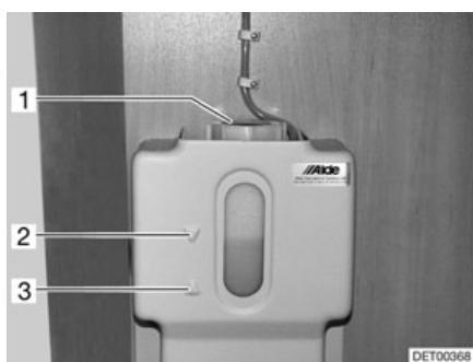
Afb. 267 Buffertank warmwaterverwarming
