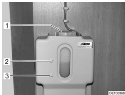
Afb. 181 Buffertank warmwaterverwarming
